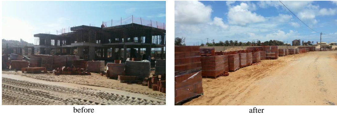
Figure 8: Before and after defining inventory areas on site
