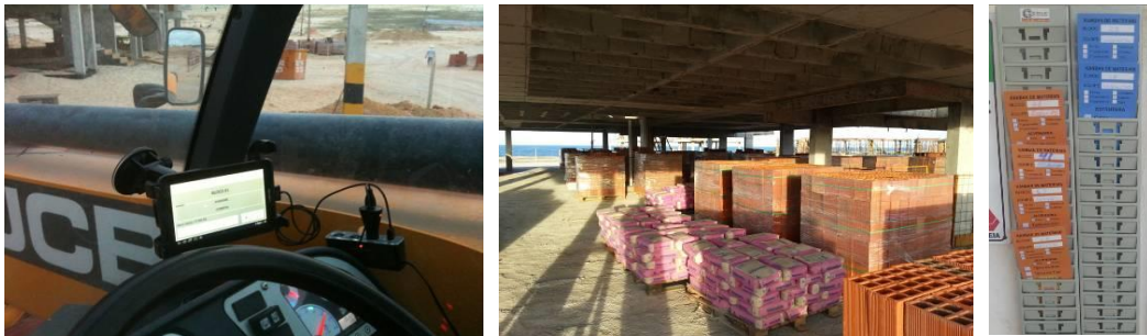
Figure 6: Tablet in a telescopic forklift, jobsite supplied and material kanban
